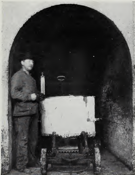
FIG. 35.—Cooking the Oil and Resin Together.
